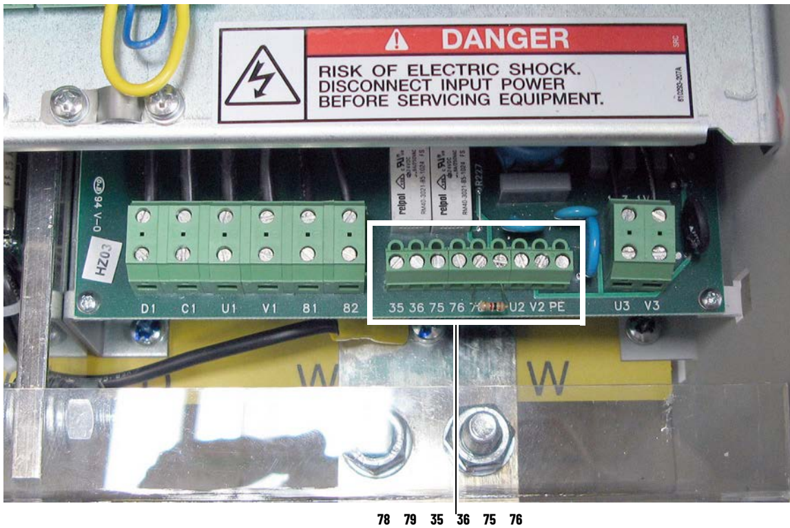
Figure 39 - 230V/460C AC Input Frame C Relay and Thermistor/Thermal Switch Terminal Block Locations
